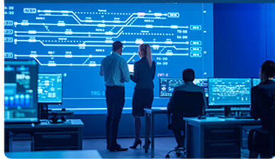
Transport Control Center
